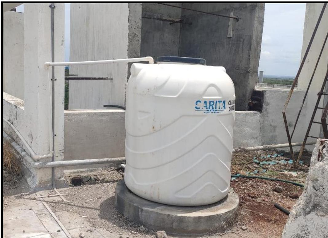
**Figure 13: Overhead Drinking Water Tank**
